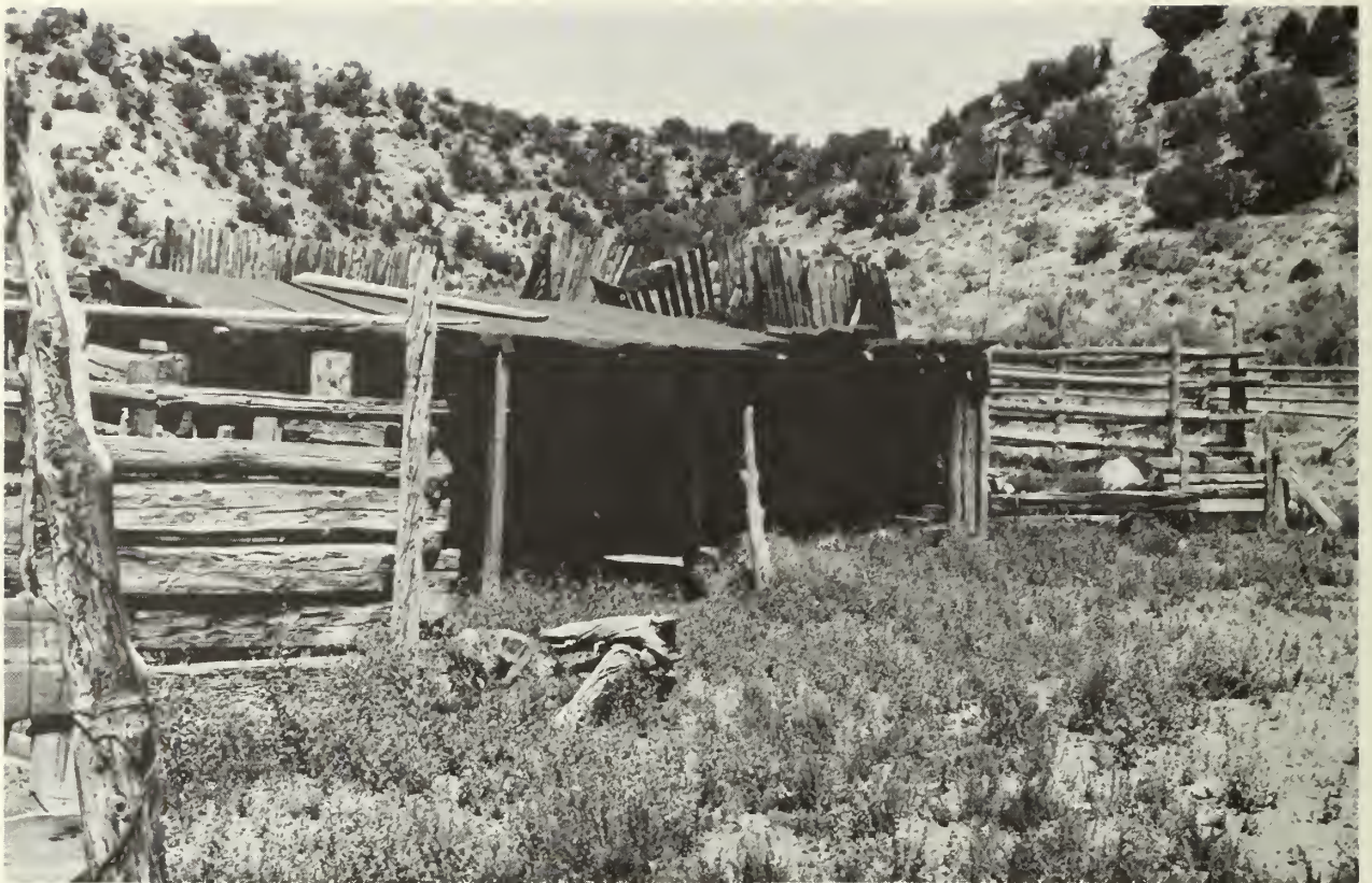
Photo 37. Jarvie corrals in 1978 showing rail tie construction. (Photo Credit: Bureau of Land Management).
